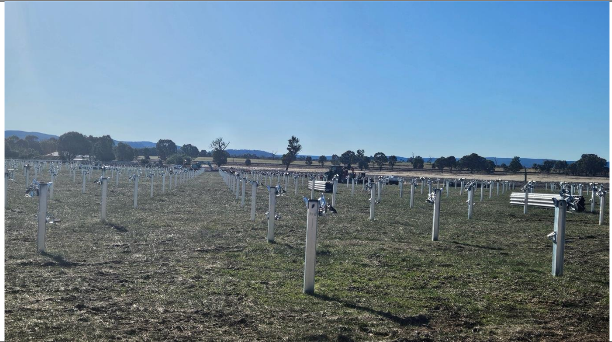
Figure 15. Mounting posts ready for frame assembly
