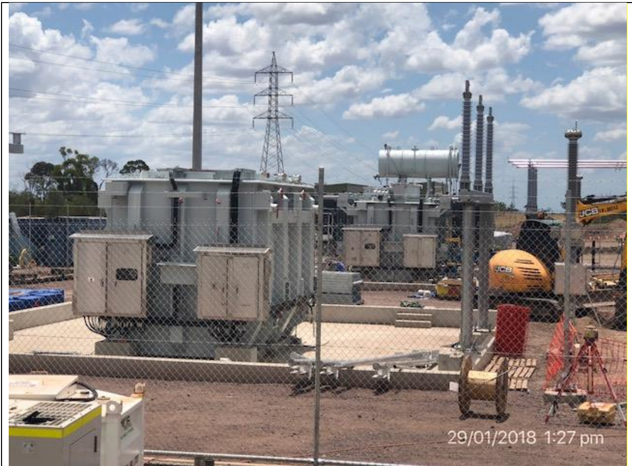
Figure 19. Indicative substation under construction
