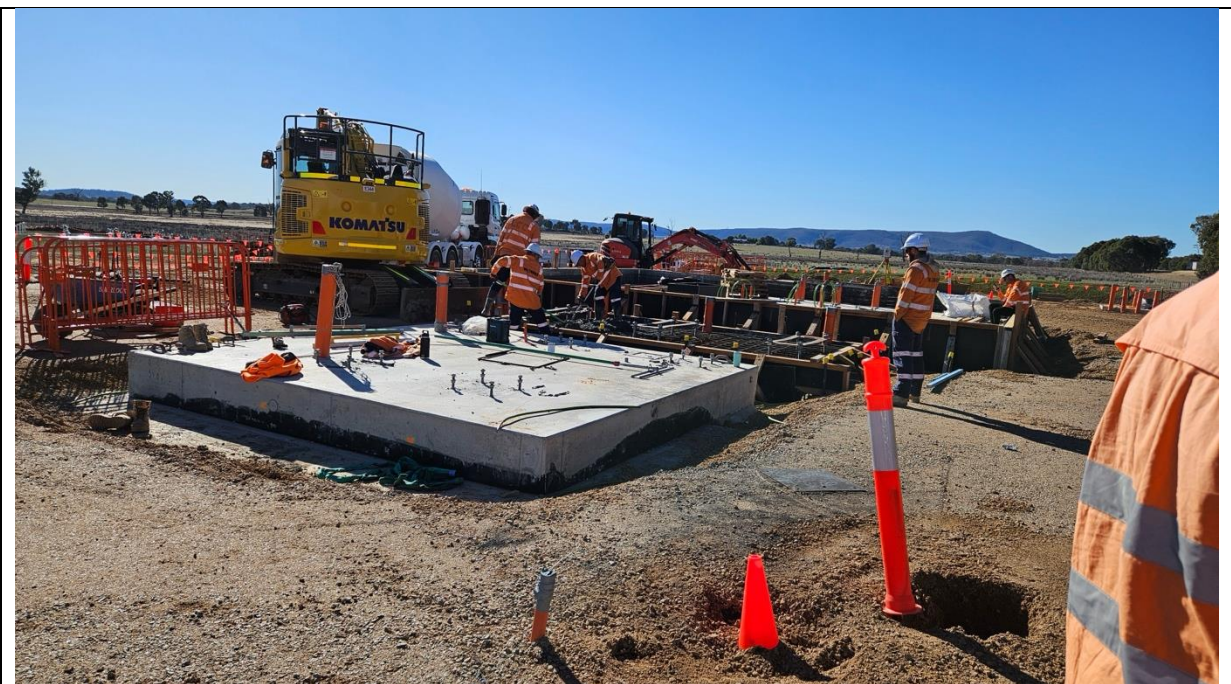
Figure 18. Power Conversion Station pad preparation
