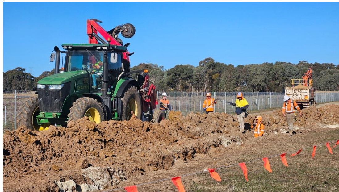
Figure 16. Installation of trenches for cabling with indicative boundary security fencing
